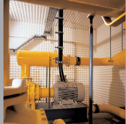
SONEXpyramid panels used in a manufacturing facility
